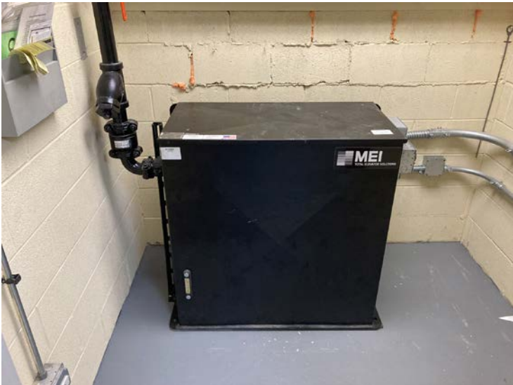
New elevator motor
