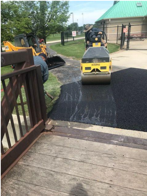
Bridge Approach repairs complete
